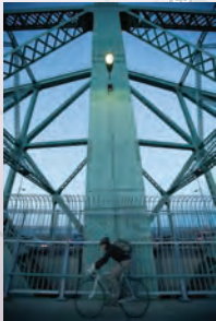
Jacques Cartier Bridge sector
