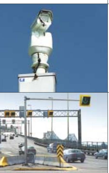
*Closed-Circuit Television Surveillance System cameras and lane signalling on the Jacques Cartier Bridge.*
