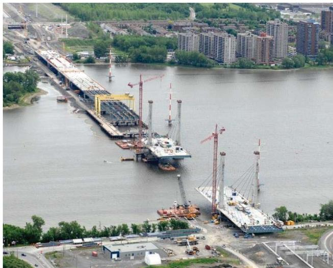
Photo 5 – Highway 25 Bridge: Overhead gantry for approach spans
