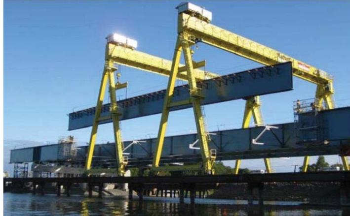
Photo 6 – Highway 25 Bridge: Two lifting gantries running on rails
