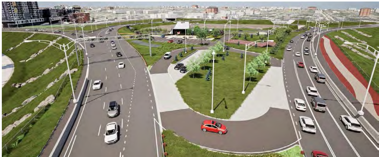
South Shore entrance to the Jacques Cartier Bridge – View toward the South Shore of the new developments
