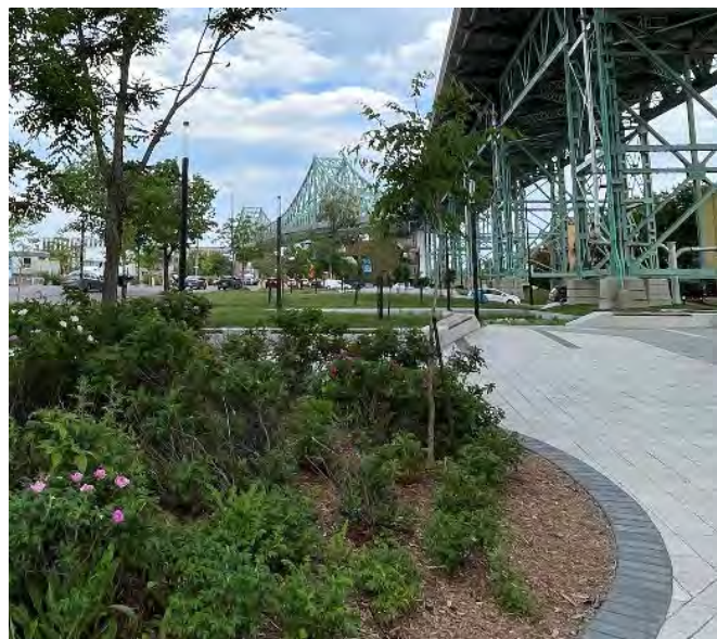
Developments under the Jacques Cartier Bridge
