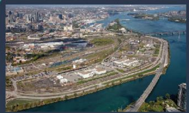
Federal section of Bonaventure Expressway
