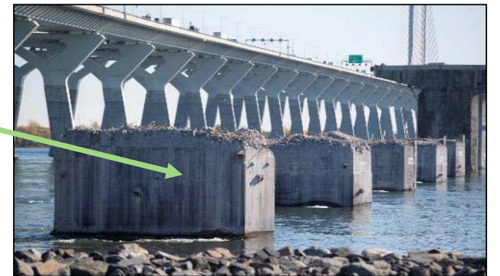
Deconstruction of piers (above water) and footings (under water)
