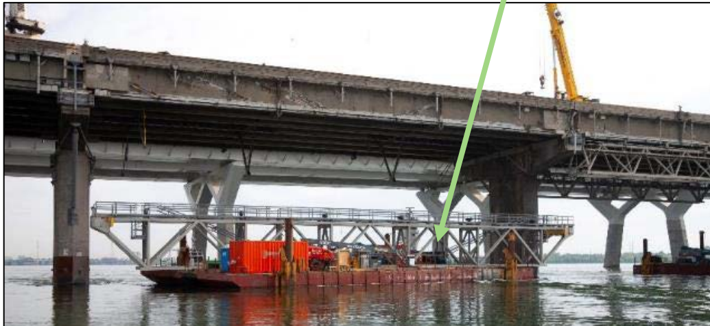
Finalization of removal of modular trusses under the marine spans
