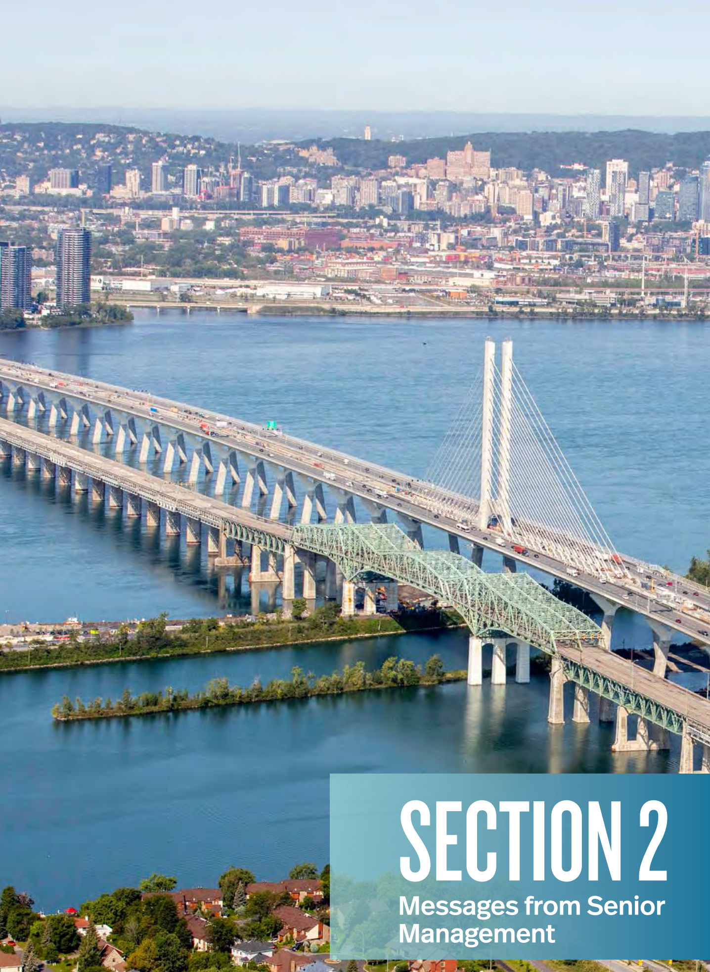
The original Champlain Bridge (left) and Samuel De Champlain Bridge (right)
