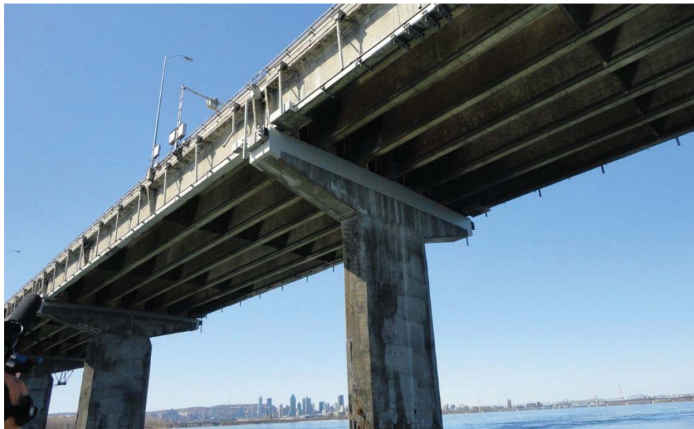
Figure A12 Typical Concrete Span in Section 5 & 7
