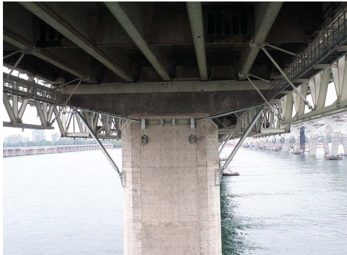
Figure 9 Pier Cap with Super-post System
