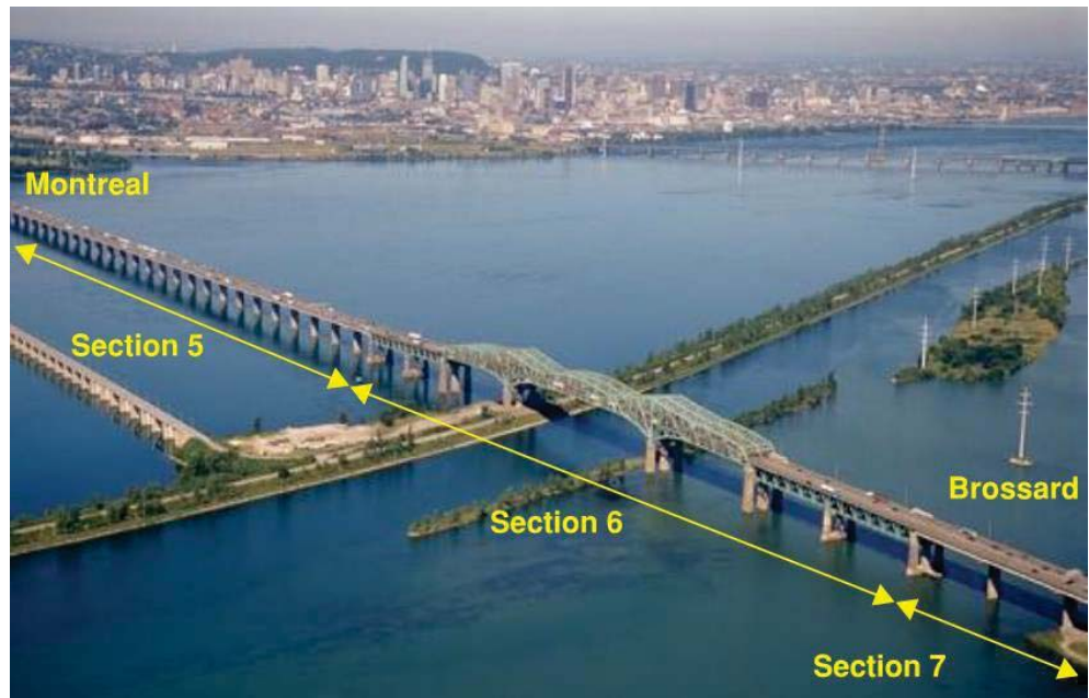
Figure A10 General View of Champlain Bridge
