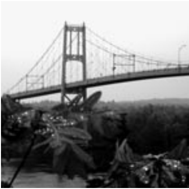
The Thousand Islands International Bridge
