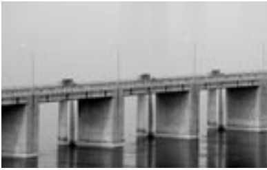
The Champlain Bridge Ice Control Structure
