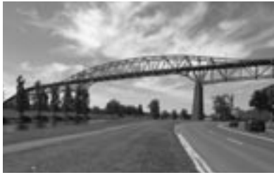
The Seaway International Bridge
