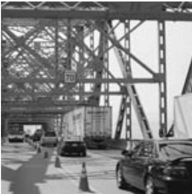
Reserved bus lane during rush hours on the Champlain Bridge in Montréal
