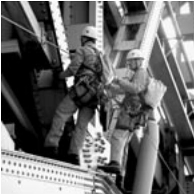
Men at work on the Champlain Bridge in Montréal
