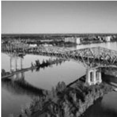
Aerial view of the Champlain Bridge in Montréal
