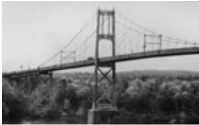
The Thousand Islands International Bridge
