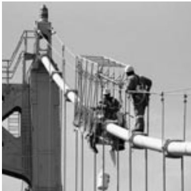
Men at work on top of the Seaway International Bridge
