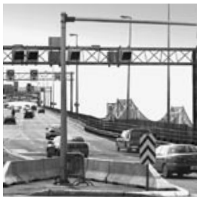
One access to the Jacques Cartier Bridge from Longueuil
