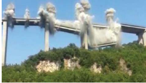
Figure 44 – Explosif – béton
