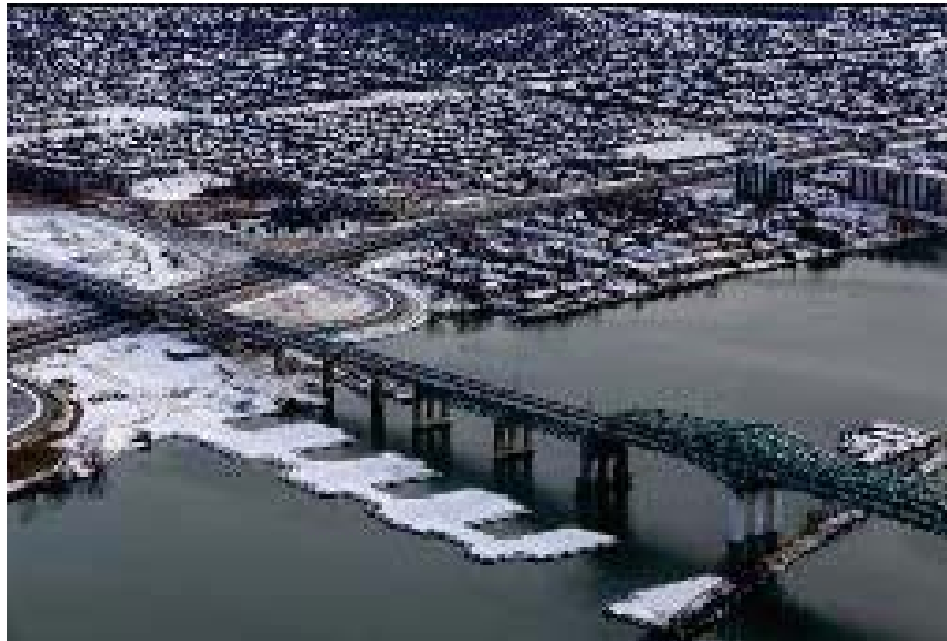
Figure 29 – Jetty on Brossard side – New Champlain Bridge (Source: newchamplain.ca)
