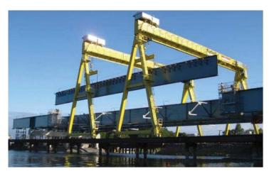
Photo 6 - Highway 25 Bridge: Two lifting gantries running on rails
