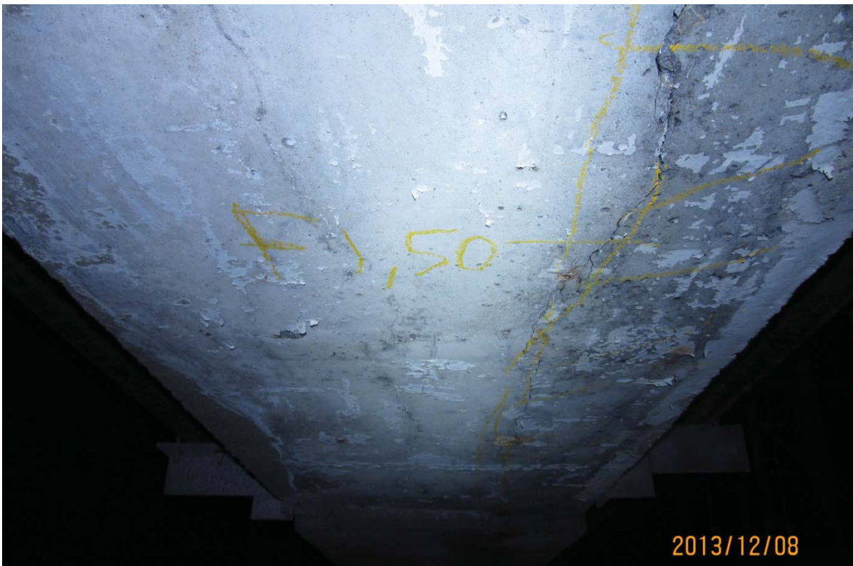
S5.PC.9W-10W.P1.d – 6673 (soffite - centre est)
