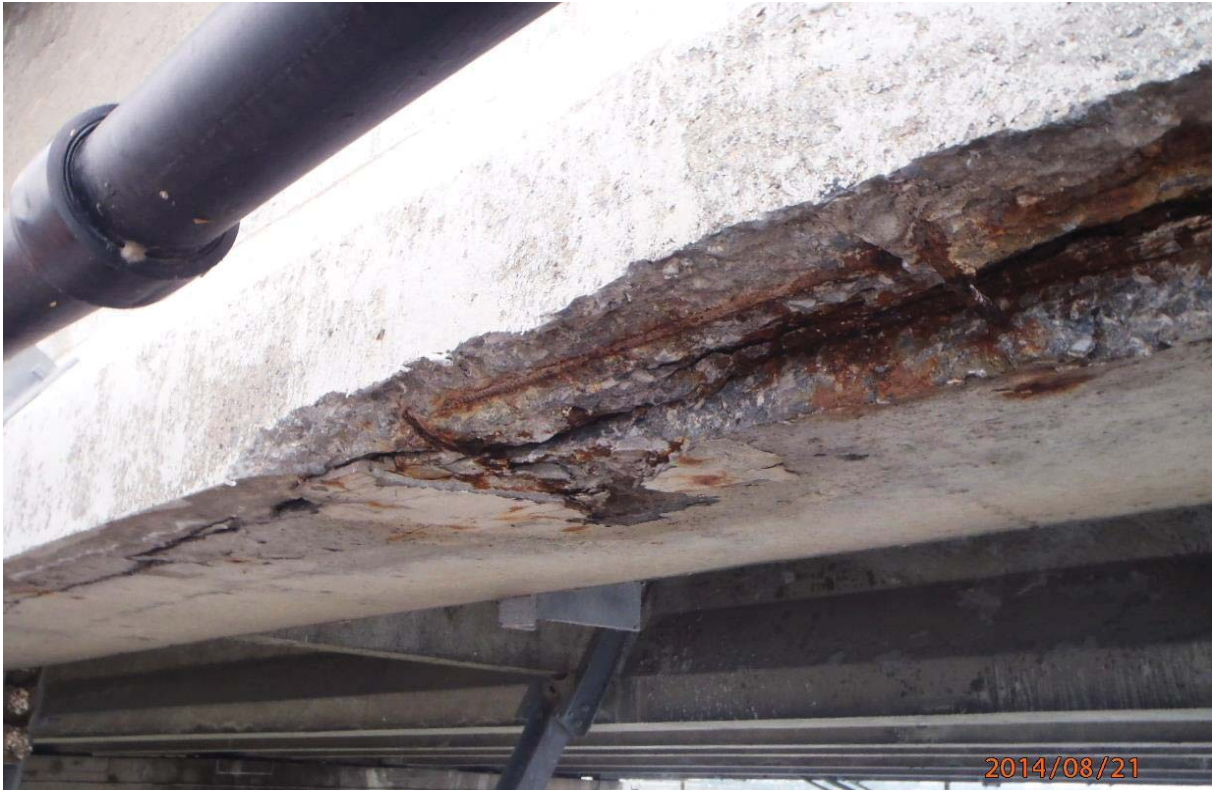
S5.PC.34W-35W.P7.g – PH.20140821_P7_34W-35W_040 (soffite – centre ouest)
