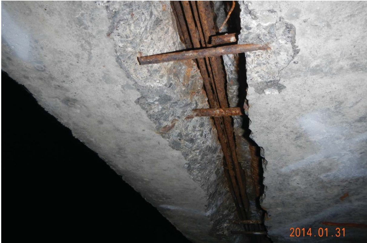
S5.PC.43W-44W.P4.e – 7481 (soffite – centre)
