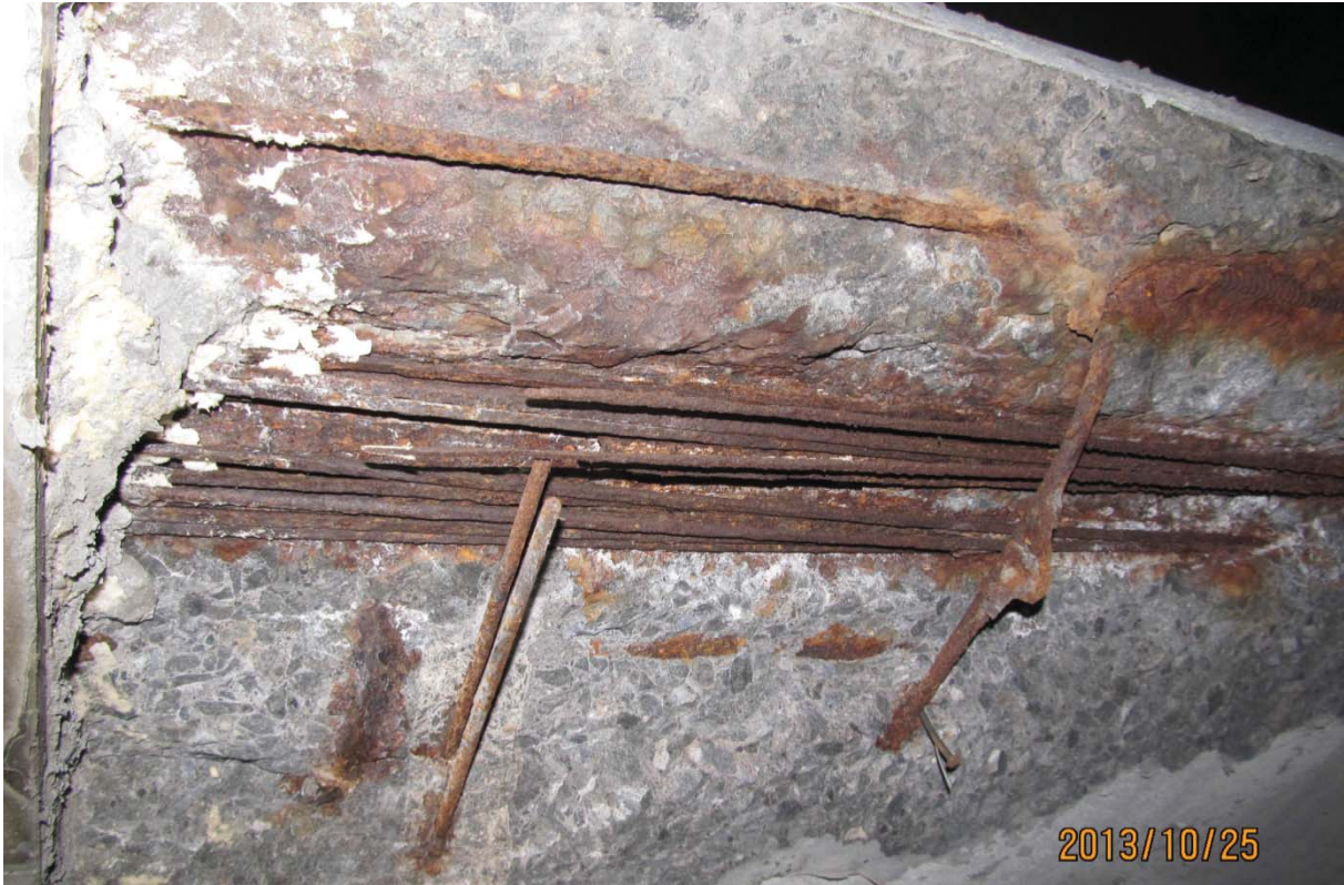
S5.PC.36W-37W.P7.e – 5924 (soffite – centre est)
