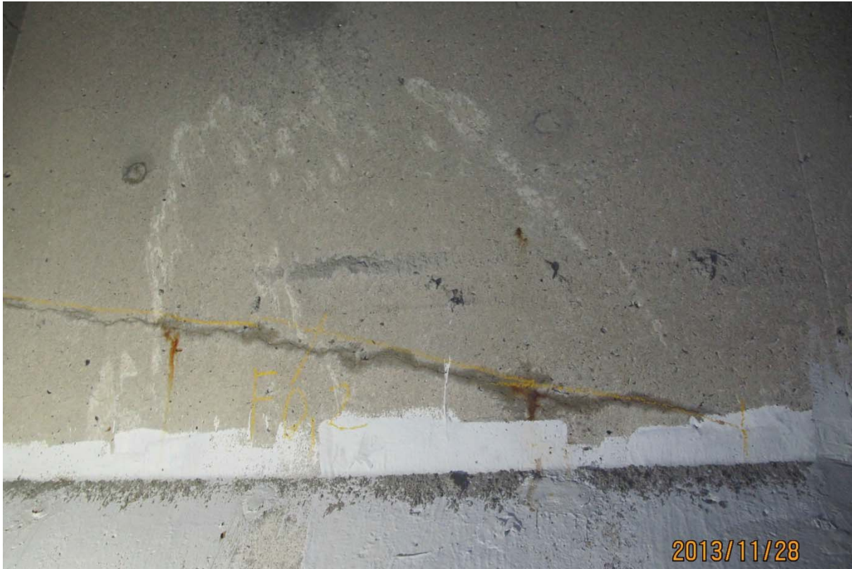
S5.PC.11W-12W.P7.c – 6489 (câble #22 – centre ouest face amont)
