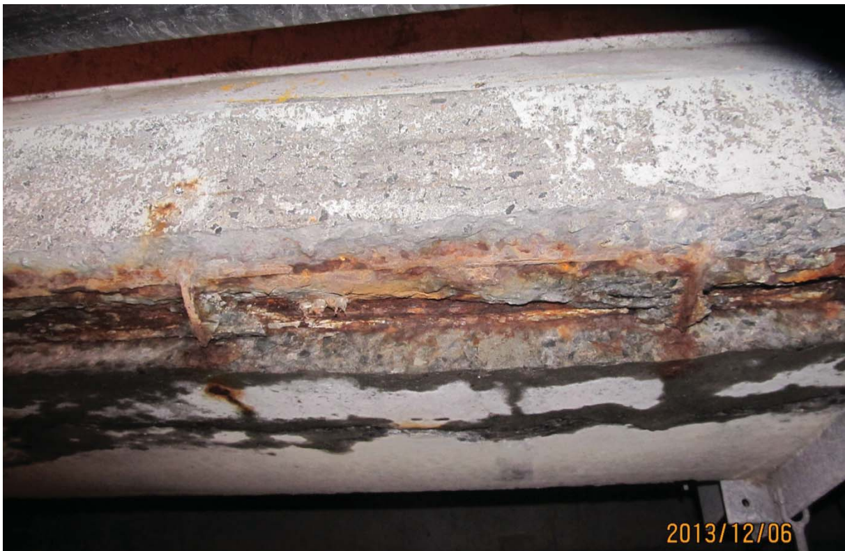
S5.PC.34W-35W.P7.f – 6622 (soffite – centre ouest)
