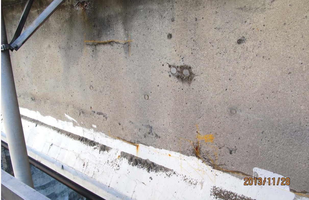
S5.PC.14W-15W.P7.e – 6477 (âme – centre ouest face amont)
