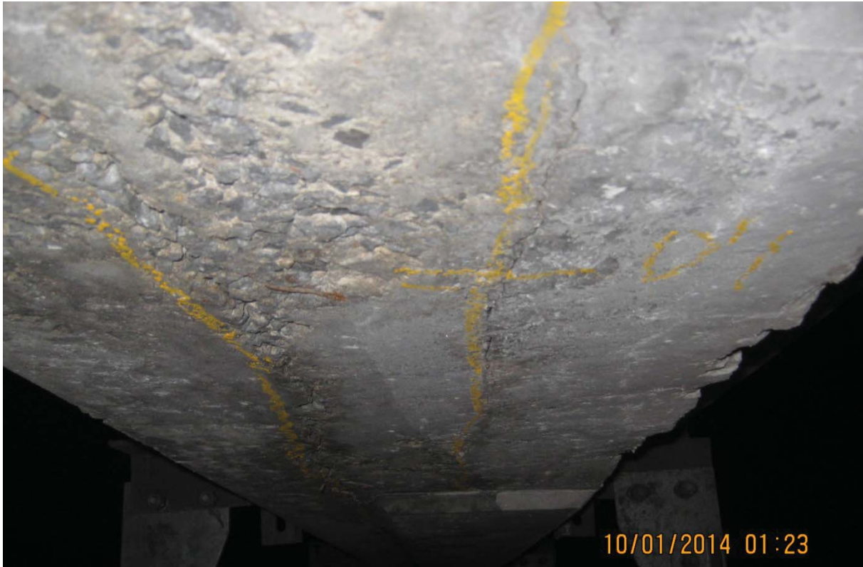
S7.PC.11E-12E.P1.a – 0260 (soffite - centre est)
