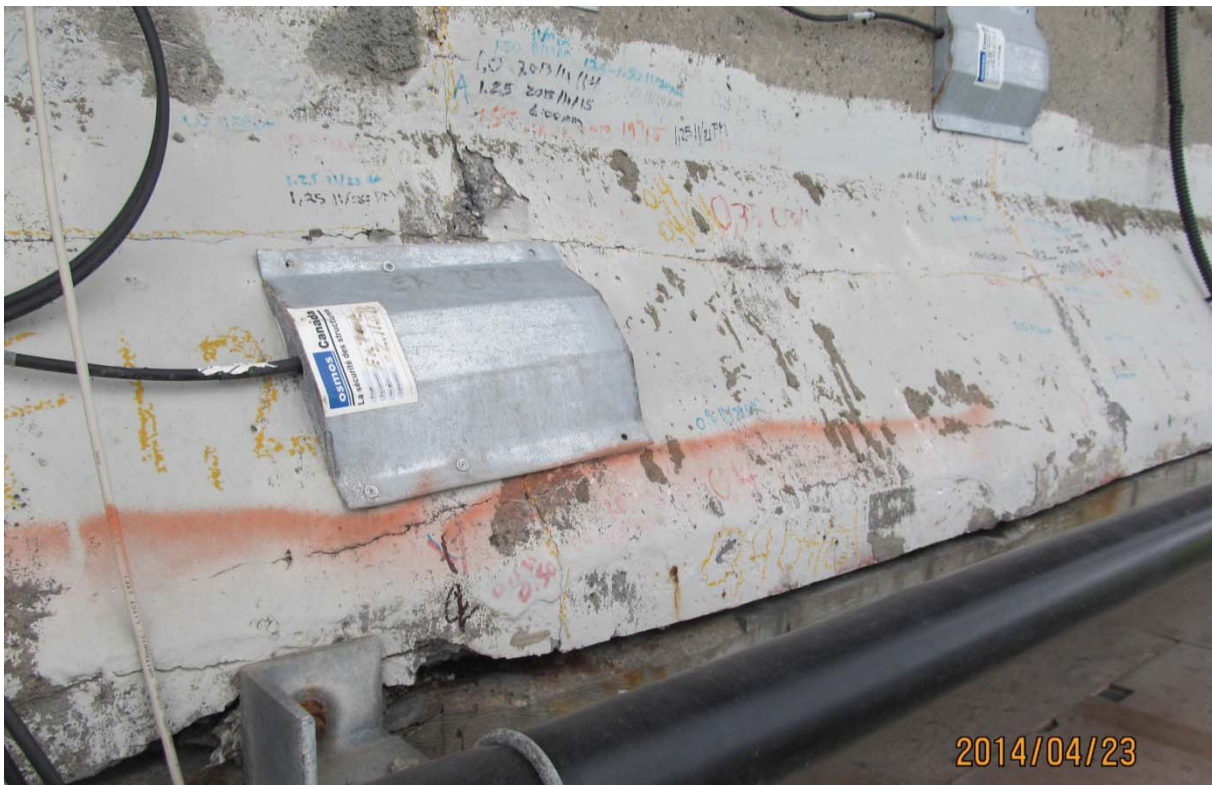
S5.PC.28W-29W.P7.m – 0444 (soffite – centre)
