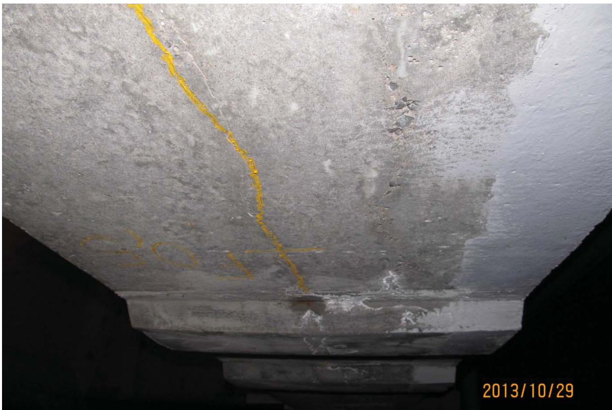
S5.PC.25W-26W.P7.f – 5971 (soffite – centre est)
