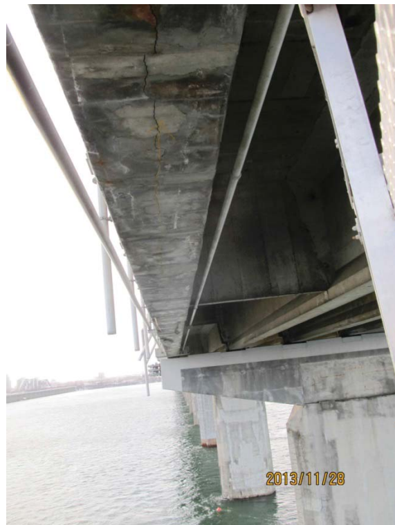
S5.PC.14W-15W.P7.m – 6479 (soffite – centre ouest)
