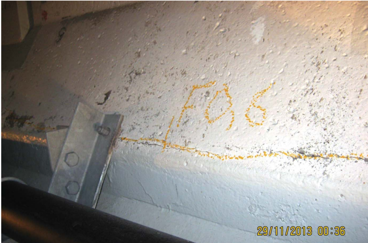
S5.PC.10W-11W.P7.c – 0110 (semelle inférieure – centre face amont)
