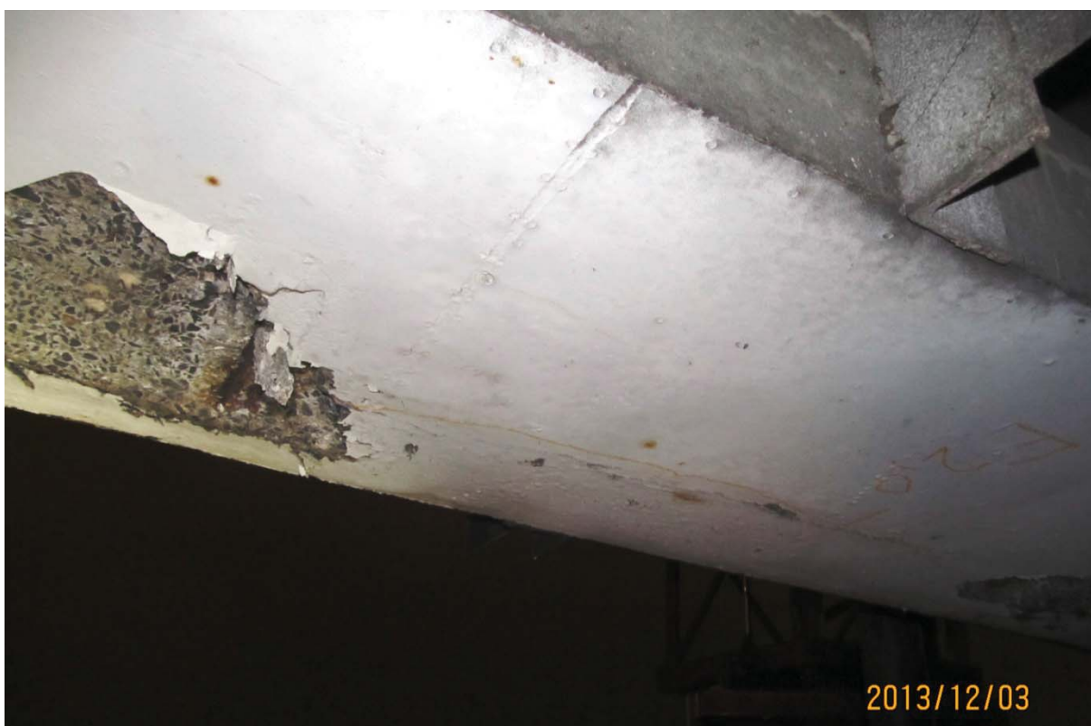
S5.PC.30W-31W.P1.h – 6552 (soffite - centre est)
