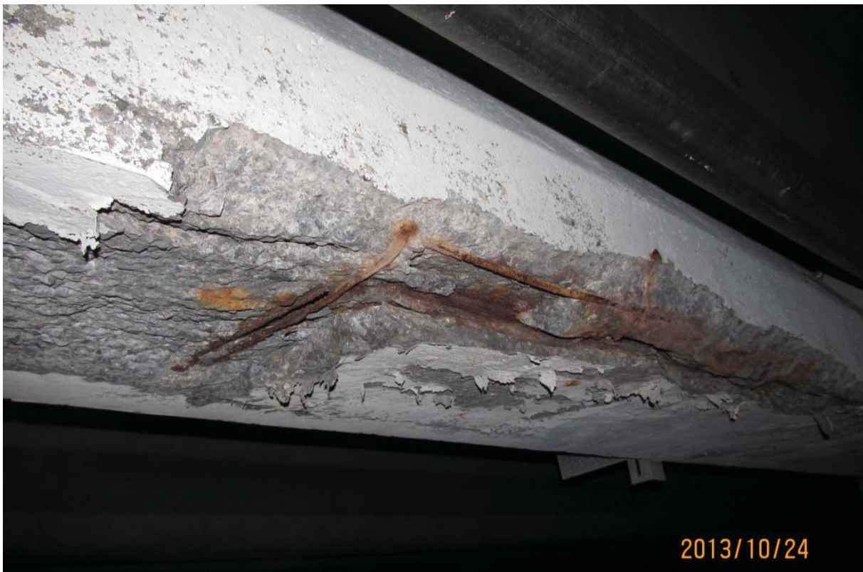
S5.PC.36W-37W.P7.f – 5920 (soffite – centre ouest)
