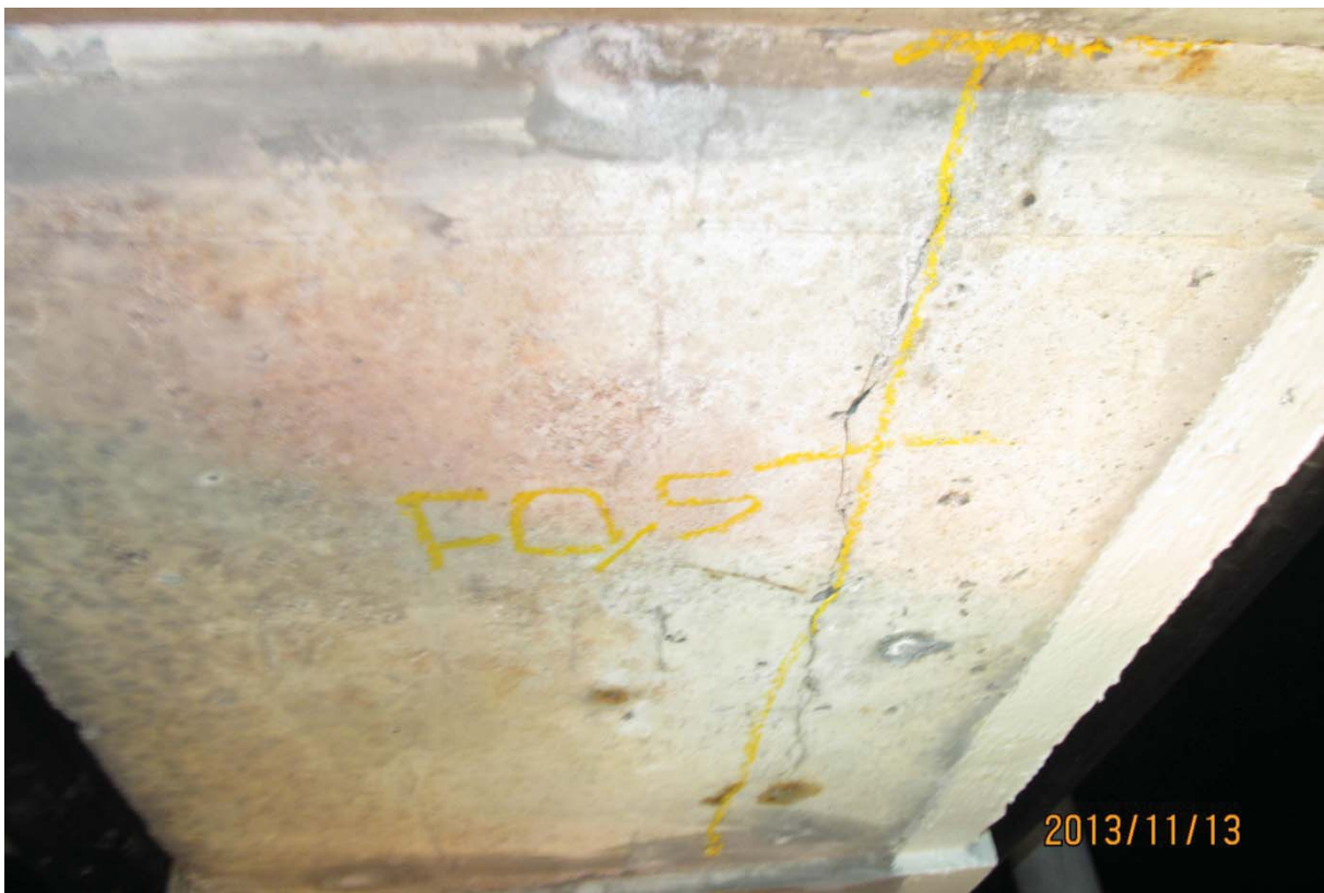
S5.PC.22W-23W.P7.b – 6279 (soffite – centre ouest)
