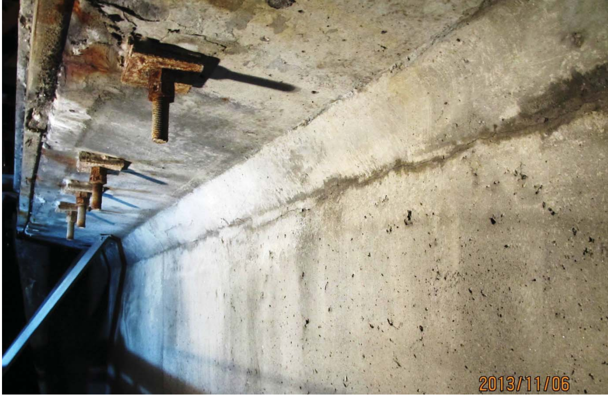
S5.PC.15W-16W.P7.c – 6151 (âme – centre ouest face amont)
