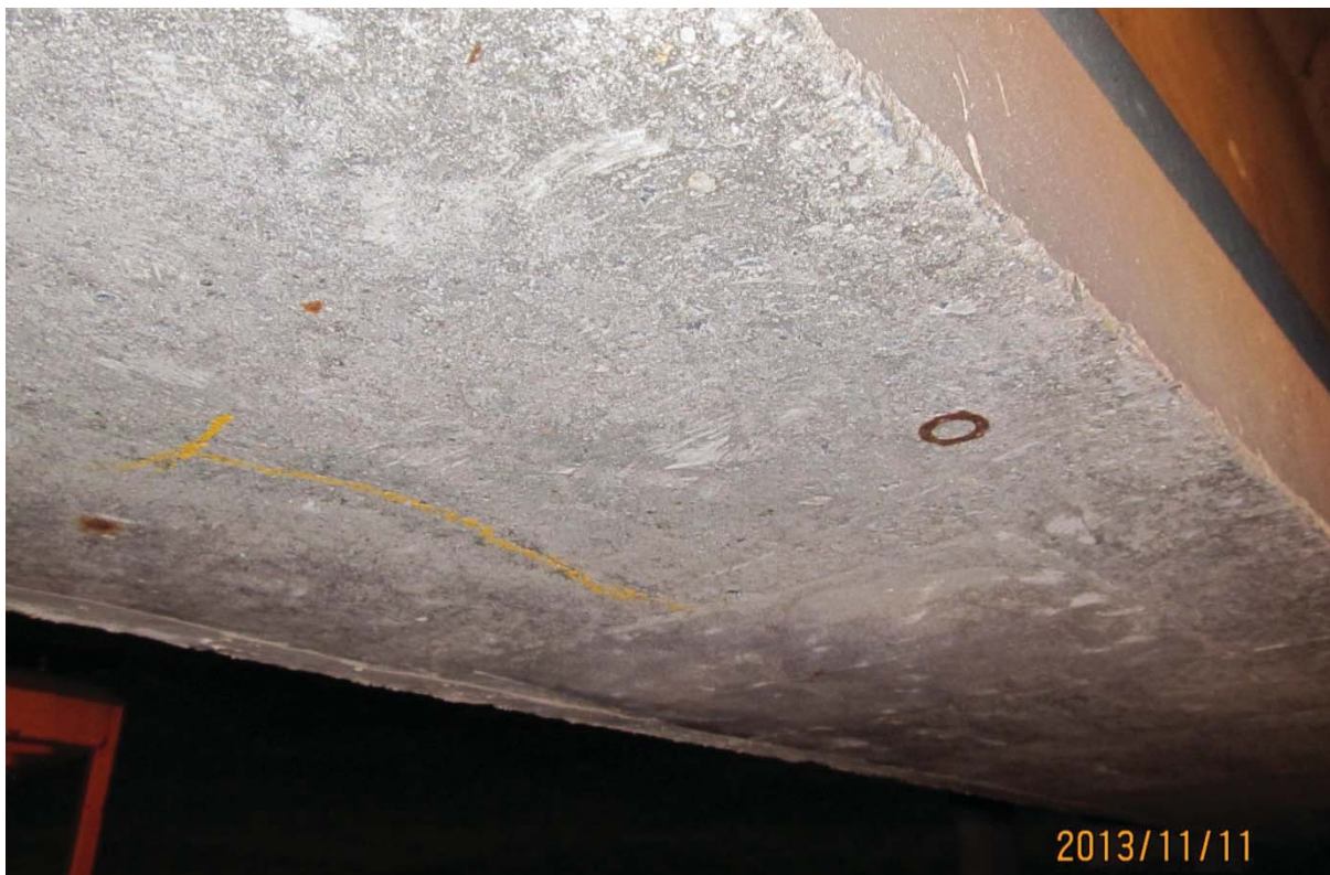
S5.PC.22W-23W.P1.a – 6221 (soffite – centre est)
