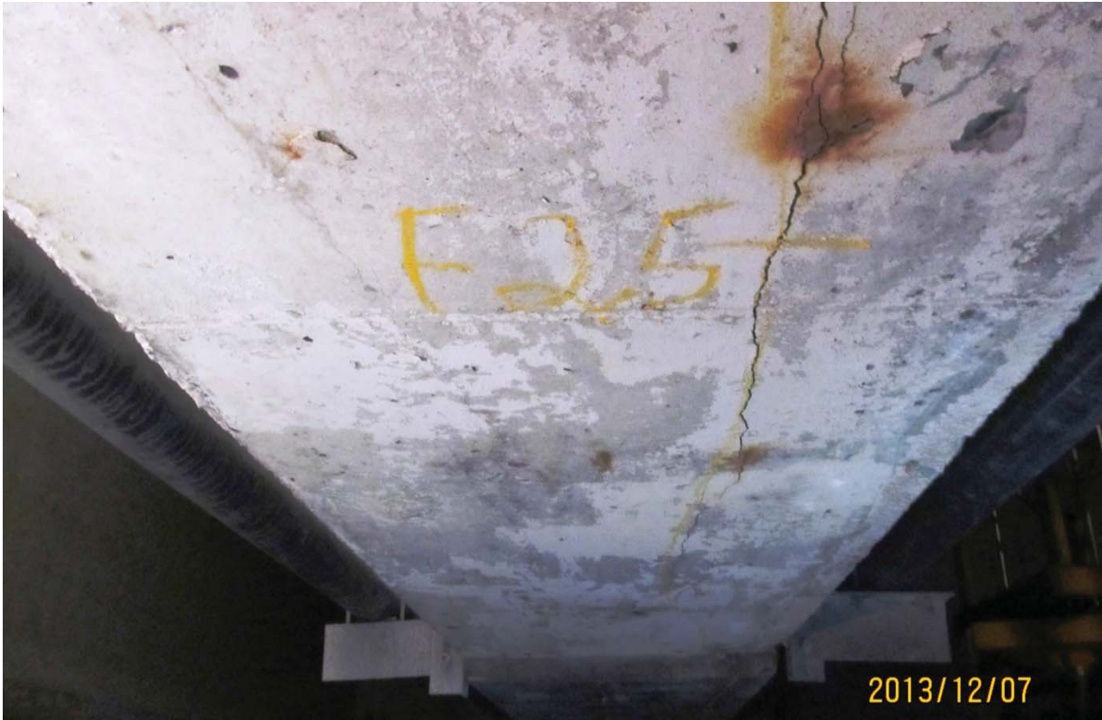
S5.PC.16W-17W.P1.c – 6654 (soffite – centre est)
