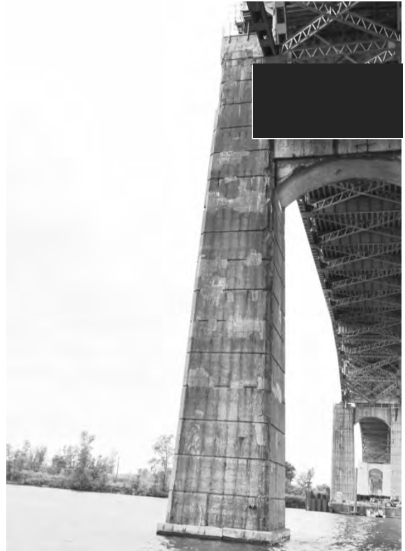
S6.PC.1.4.b – 5236 – Pile 2E (face est)
