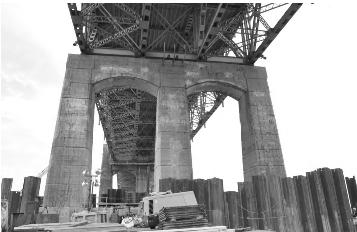
S6.PC.1.5.a – 5276 – Pile 3E (face est)
