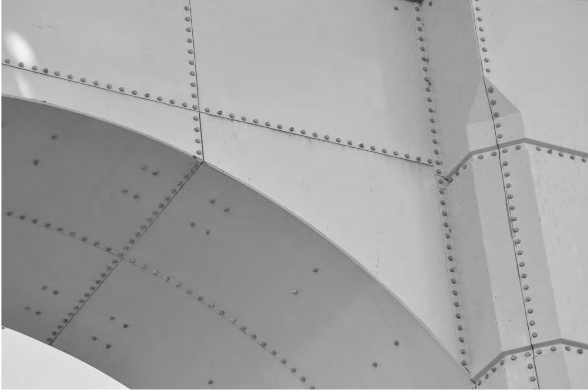
S6.PC.1.2.c – 3554 – Pile 1W (face ouest)
