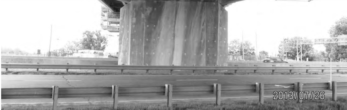
S7.PC.2.3.a – 5467 – Pile 11E
