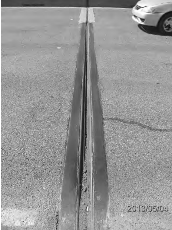
S7.PC.3.3.a – 4031 – Joint 12E (Amont)
