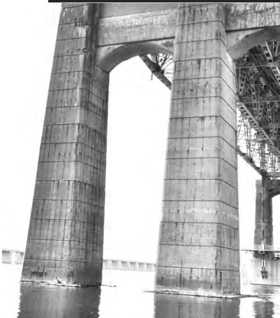
S6.PC.1.1.b – 5129 – Pile 2W (face est)
