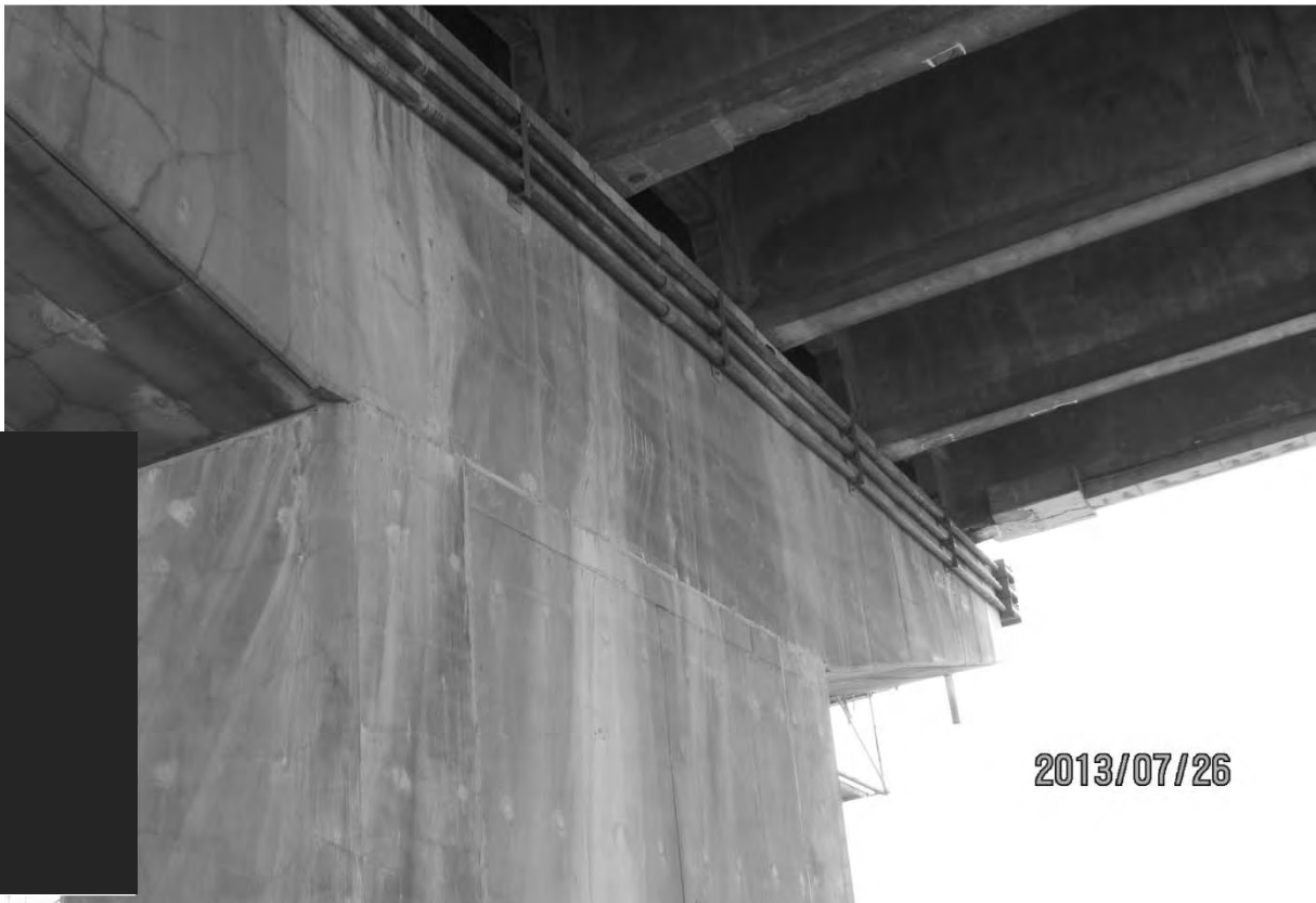
S7.PC.2.3.b – 5473 – Pile 11E
