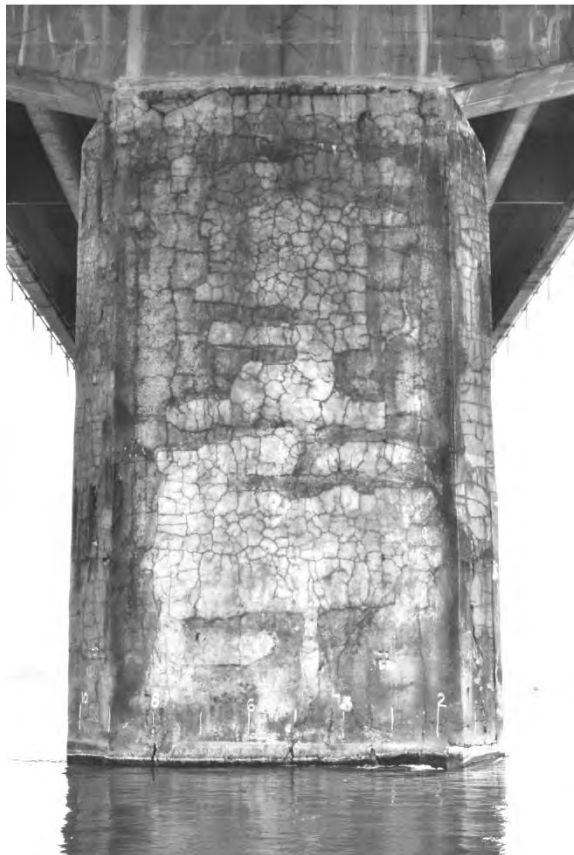
S5.PC.1.19.b – 4860 – Pile 25W (face ouest)
