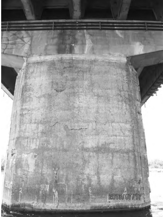
S5.PC.1.8.a – 4770 – Pile 36W (face est)
