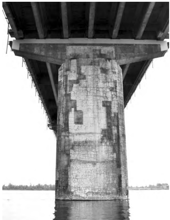
S5.PC.1.29.b – 4974 – Pile 15W (face ouest)
