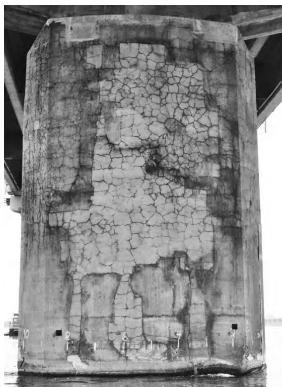
S5.PC.1.16.b – 4825 – Pile 28W (face ouest)
