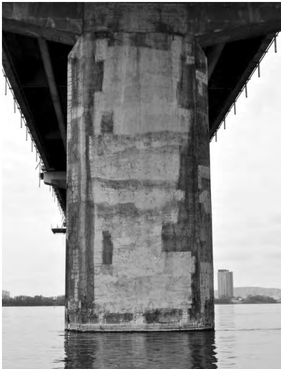
S5.PC.1.29.a – 4983 – Pile 15W (face est)
