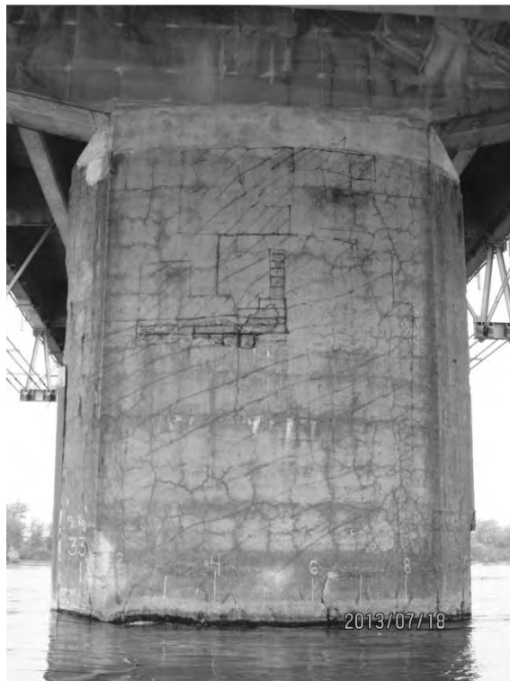
S5.PC.1.11.a – 4806 – Pile 33W (face est)
