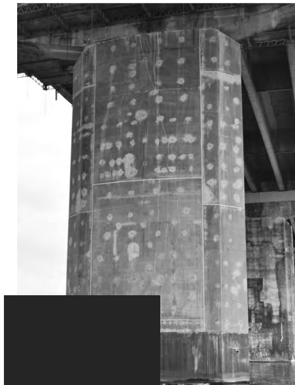
S5.PC.1.27.b – 4955 – Pile 17W (face ouest)
