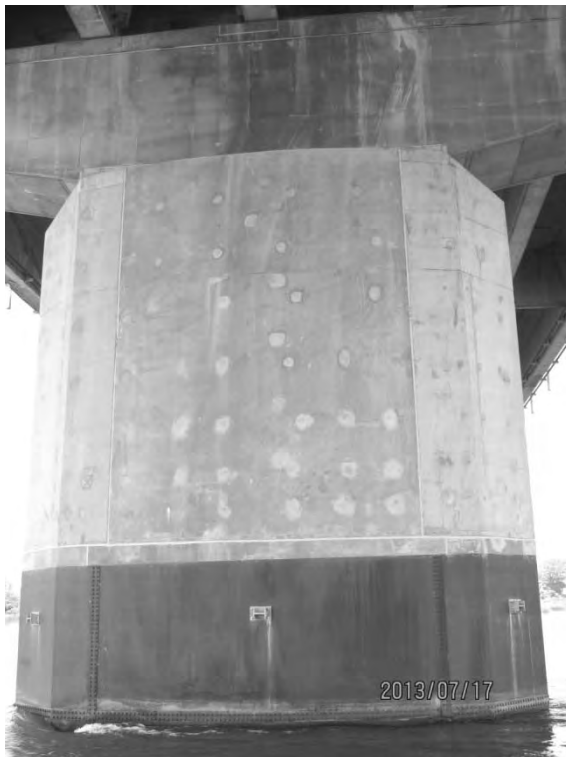
S5.PC.1.9.a – 4779 – Pile 35W (face est)
