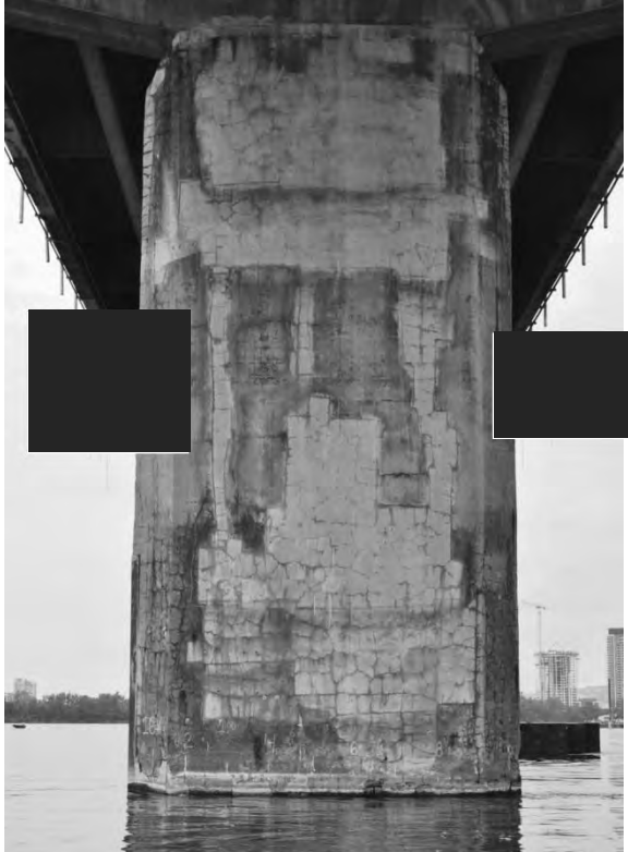
S5.PC.1.28.a – 4972 – Pile 16W (face est)
