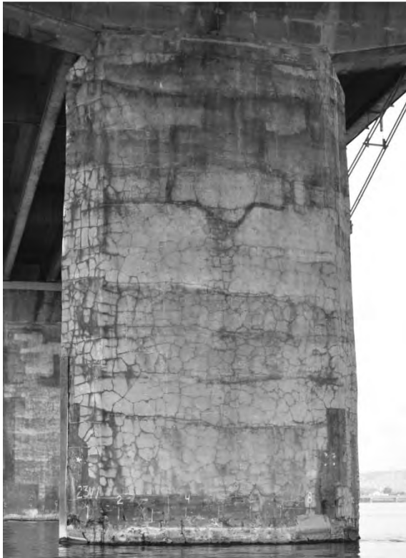
S5.PC.1.21.a – 4894 – Pile 23W (face est)
