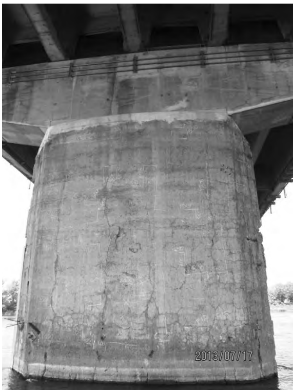
S5.PC.1.7.a – 4757 – Pile 37W (face est)
