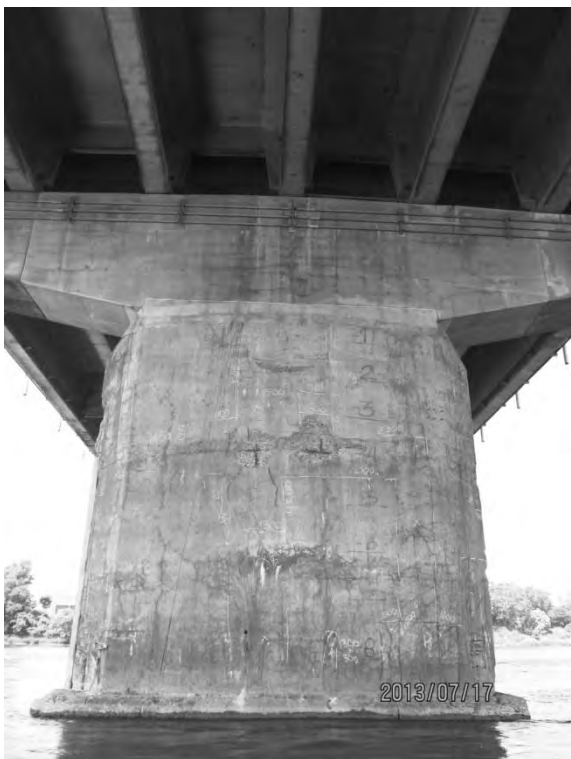
S5.PC.1.6.a – 4748 – Pile 38W (face est)
