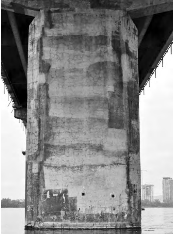
S5.PC.1.26.a – 4951 – Pile 18W (face est)
