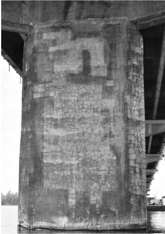
S5.PC.1.20.a – 4880 – Pile 24W (face est)
