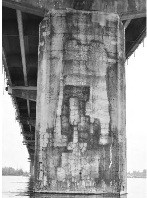
S5.PC.1.28.b – 4965 – Pile 16W (face ouest)
