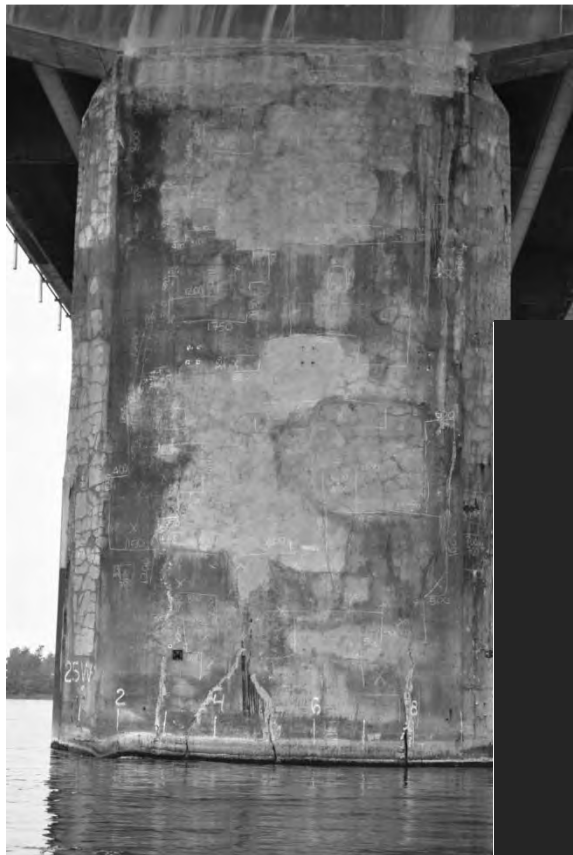
S5.PC.1.19.a – 4867 – Pile 25W (face est)
