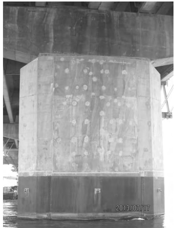
S5.PC.1.9.b – 4773 – Pile 35W (face ouest)
