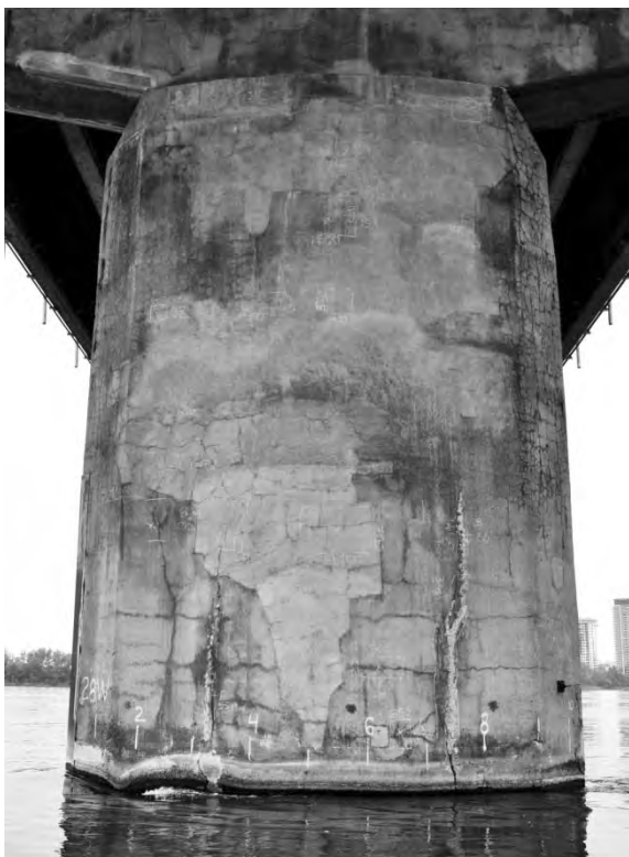
S5.PC.1.16.a – 4831 – Pile 28W (face est)
