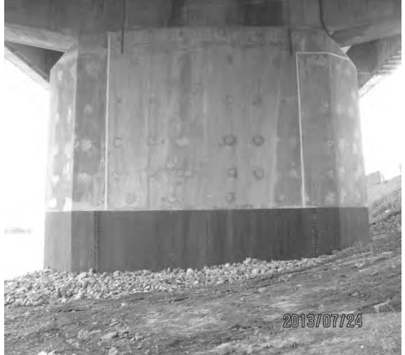
S5.PC.1.3.b – 1698 – Pile 41W (face est)
