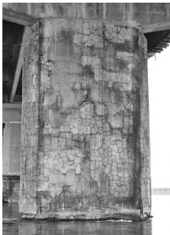
S5.PC.1.17.b – 4840 – Pile 27W (face ouest)
