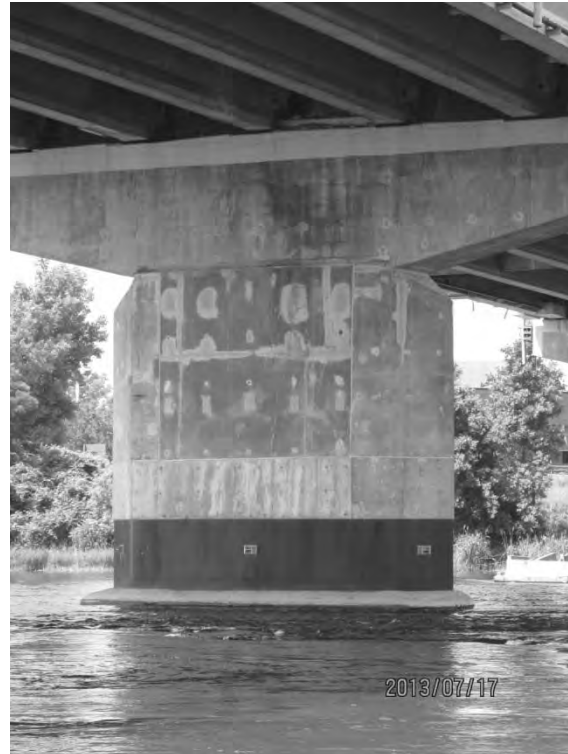
S5.PC.1.5 – 4741 – Pile 39W (face est)
