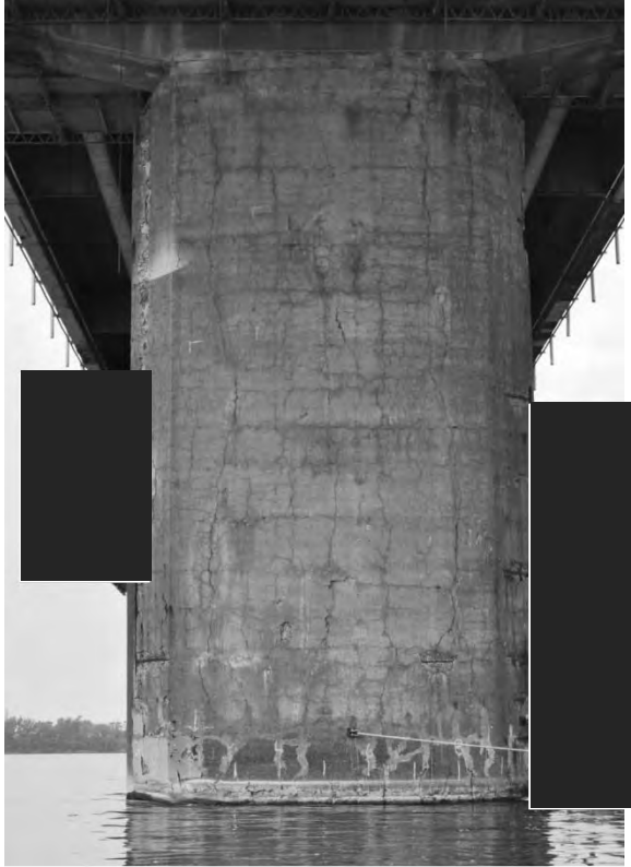
S5.PC.1.24.a – 4925 – Pile 20W (face est)
