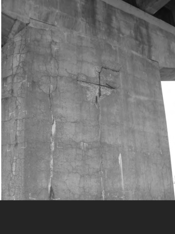
S5.PC.1.4.a – 1696 – Pile 40W (face est)
