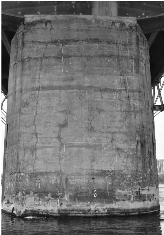
S5.PC.1.13.a – 4789 – Pile 31W (face est)
