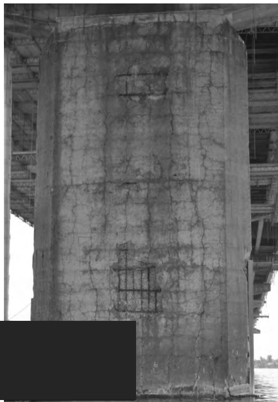
S5.PC.1.22.b – 4897 – Pile 22W (face ouest)
