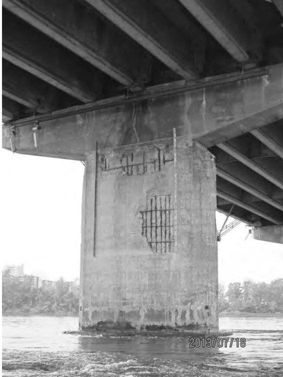
S5.PC.1.10.a – 4799 – Pile 34W (face est)
