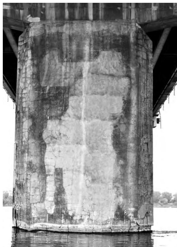
S5.PC.1.17.a – 4847 – Pile 27W (face est)
