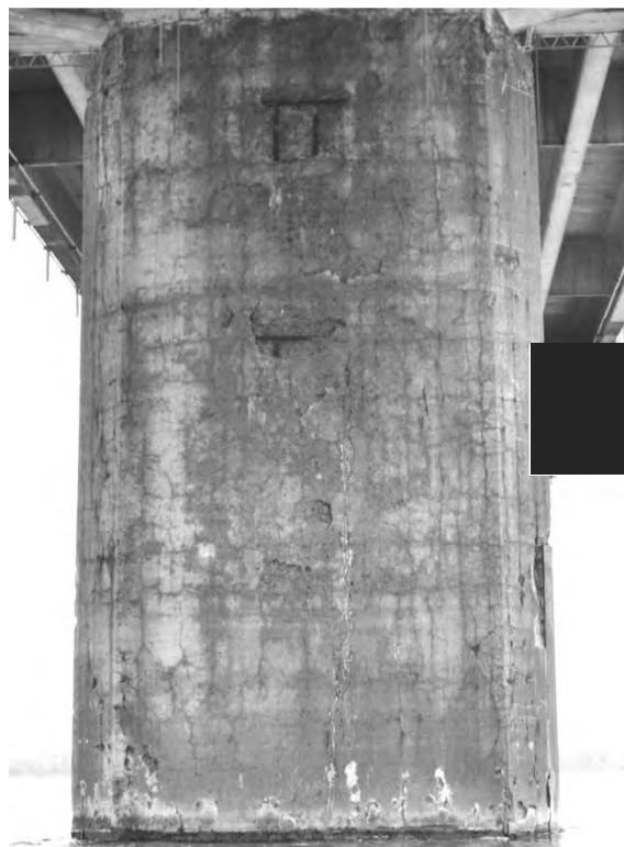
S5.PC.1.23.b – 4907 – Pile 21W (face ouest)
