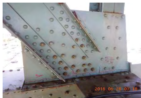
Photo plaque aval, face extérieure:
