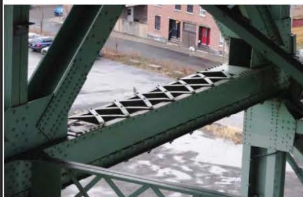
Photo 1: Corde inférieure JC_8_20151214_3682
