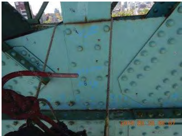
Photo plaque aval, face extérieure:
