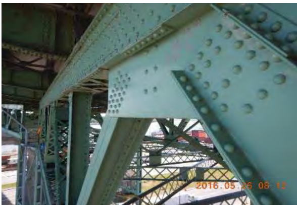
Photo plaque aval, face extérieure:
