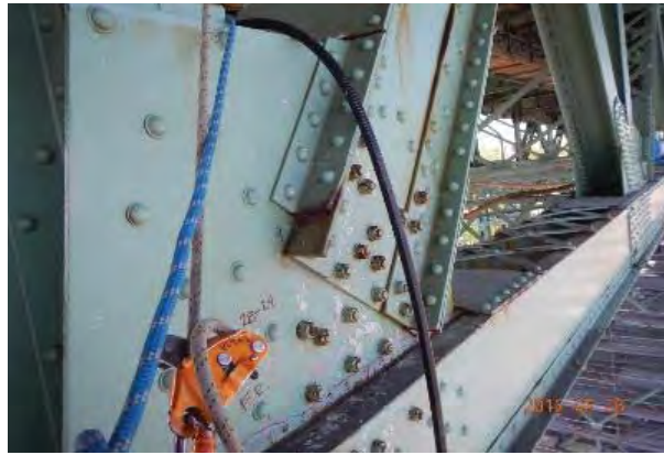
Photo plaque aval, face extérieure:
