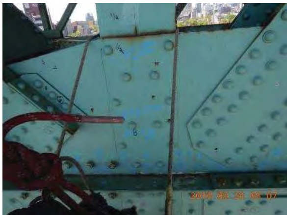
Photo plaque aval, face extérieure:
