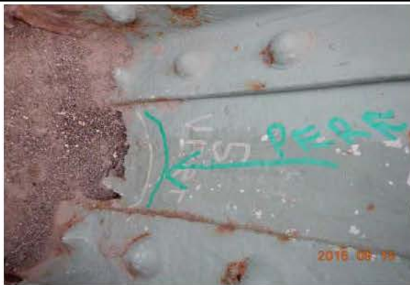
Photo 1: Perforation JC_5_160915_8677
