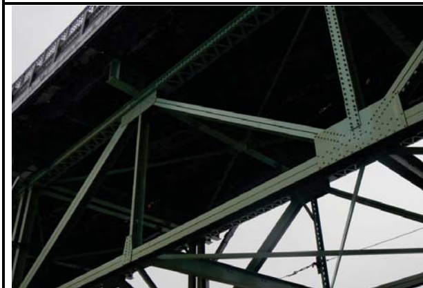
Photo 1: Corde inf. L1-L2, face sud JC_5_20160126_JM_8549
