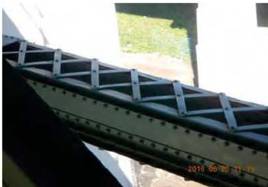
Photo 1: Corde inférieure JC_4_160823_JM_0771
