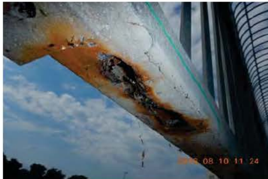
Photo 1: Perforation lisse inf.
