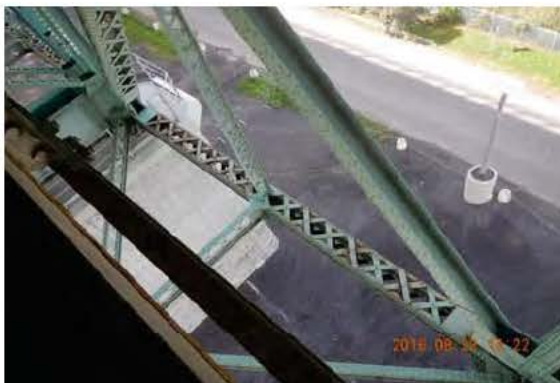
Photo 1: Corde inférieure JC_4_160822_JM_0635
