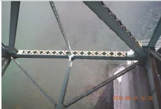
Photo 1: Corde inférieure L8-L10 JC_4_160822_JM_0608
