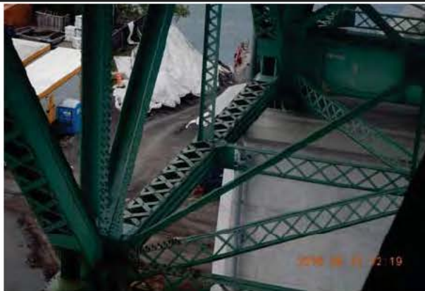
Photo 1: Corde inférieure JC_4_160822_JM_0534
