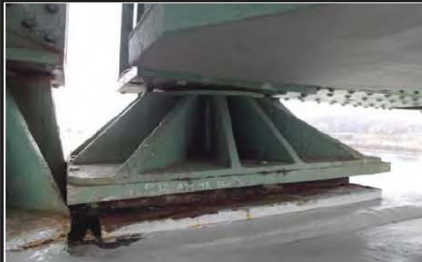
Photo 1: App. appui mobile JC_4_20151209_3367
