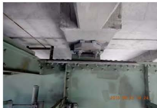
Photo 2: App. Appui platine U0 JC_4_160823_JM_0727
