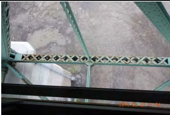
Photo 1: Corde inférieure JC_4_160822_JM_0519
