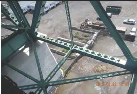
Photo 1: Corde inférieure JC_4_160822_JM_0545
