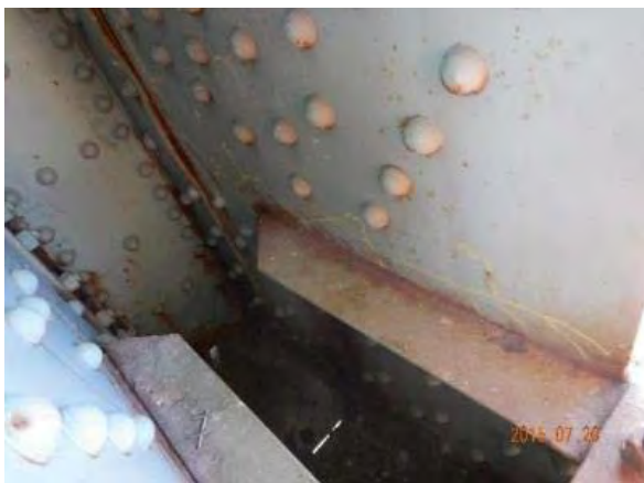
Photo plaque amont, face aval :
