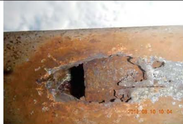
Photo 2: Perforation JC_4_160810_JM_0119
