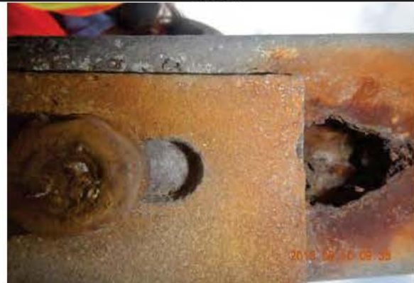
Photo 2: Perforation JC_4_160810_JM_0111
