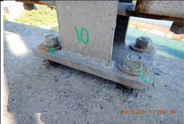
Photo 2: Extr. ancrages court.
