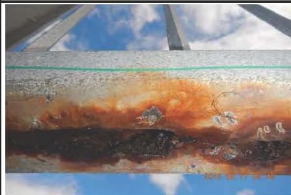
Photo 1: Perforation JC_4_160817_JM_0386
