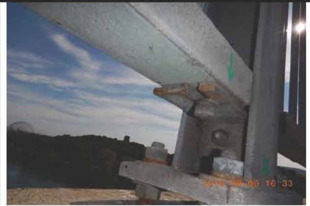
Photo 2: Dist. rive insuffisante JC_4_160809_EM_8472
