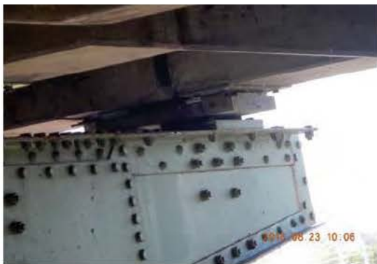
Photo 1: App. Appui platine U0 JC_4_160823_JM_0710
