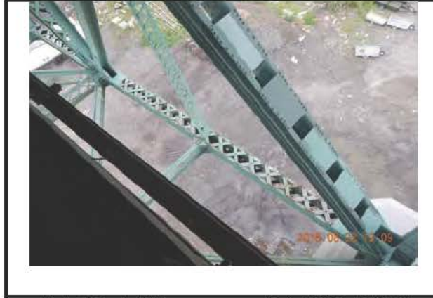
Photo 1: Corde inférieure JC_4_160822_JM_0527
