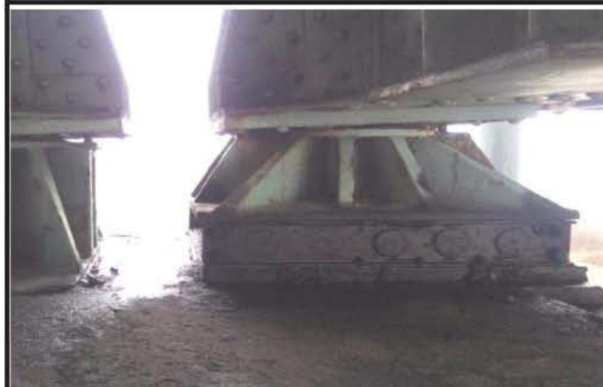
Photo 1: App. appui mobile N-O JC 2 20151127 MF 9403
