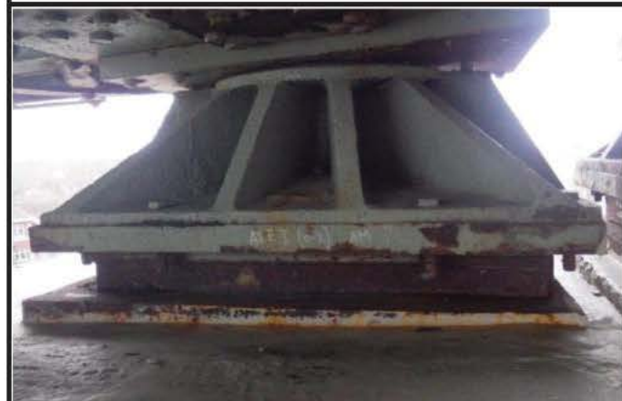
Photo 1: App. Appui mobile S-O JC_2_20151127_MF_9354
