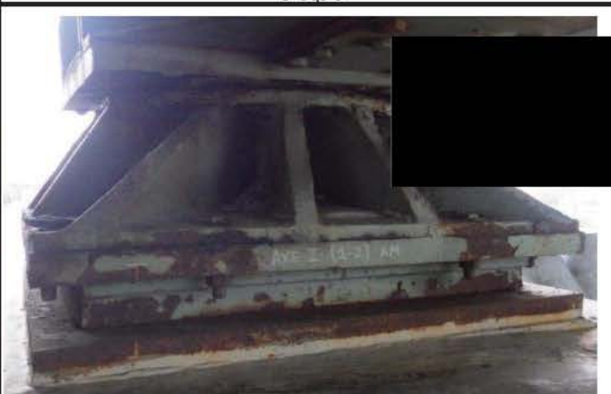
Photo 2: App. Appui mobile N-O JC_2_20151127_MF_9355
