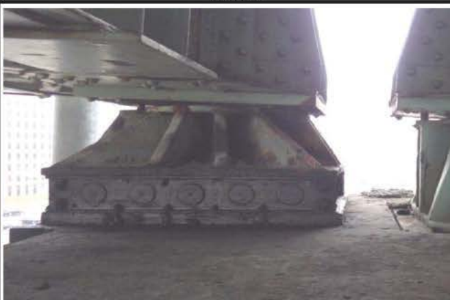
Photo 2: App. appui mobile N-E JC 2 20151127 MF 9404
